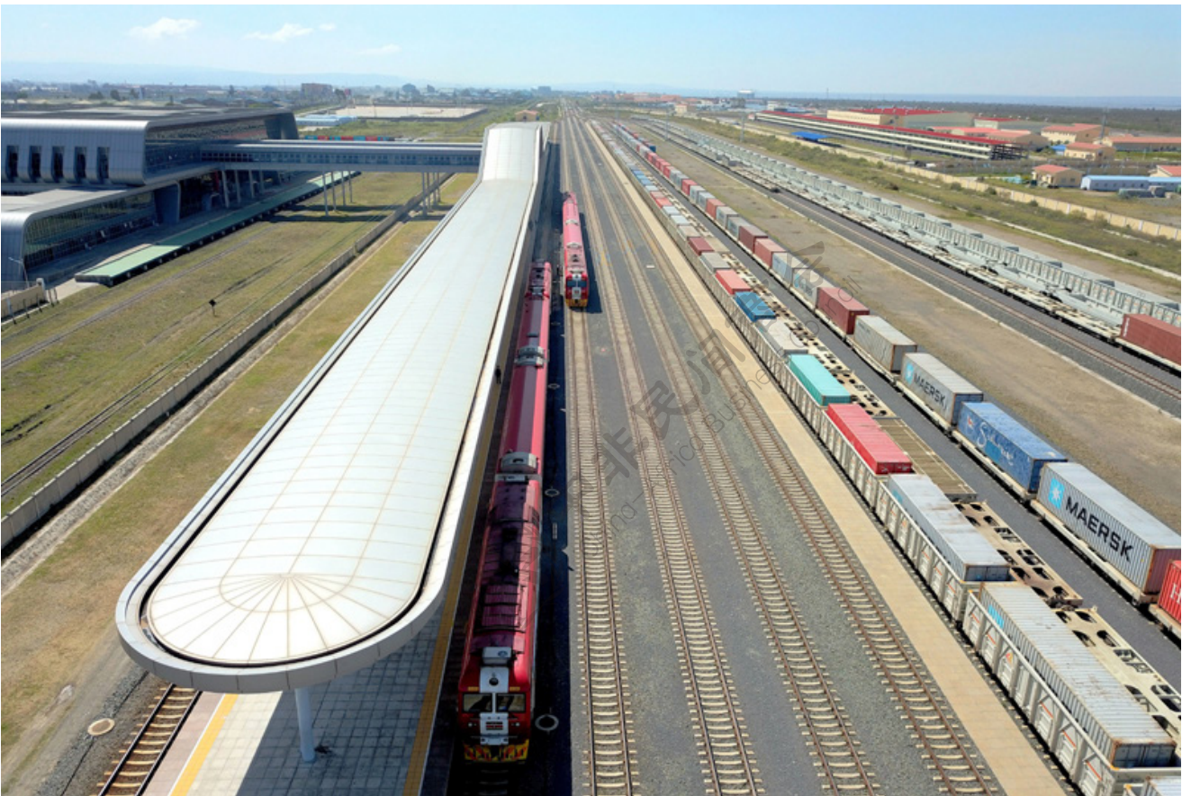
Figure 12 Nairobi-Malaba Railway Phase I opened to traffic
